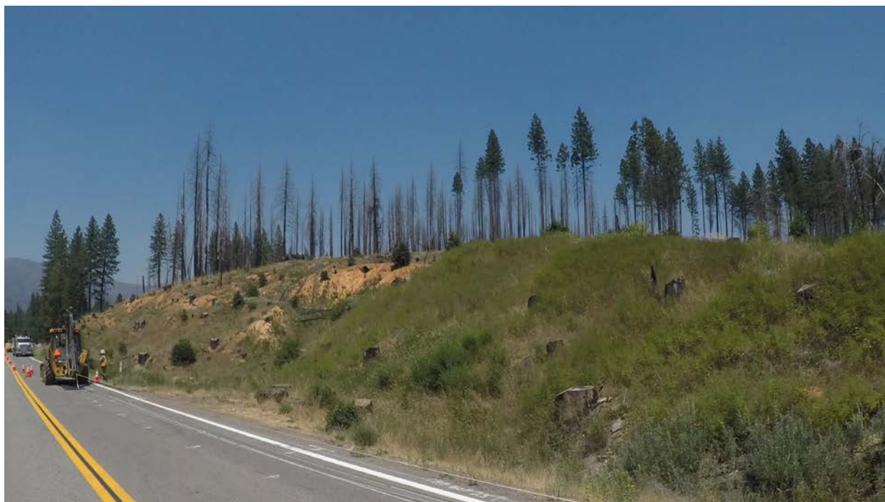
Figure 14: Shrubby vegetation regrowth off Highway 89 immediately outside of Greenville.
