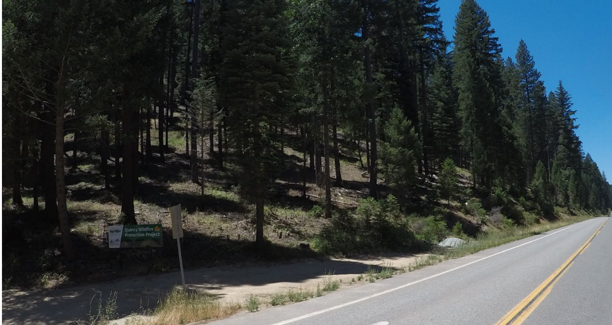
Figure 21: Treated roadside hillside on Bucks Lake Road, outside of Quincy.
